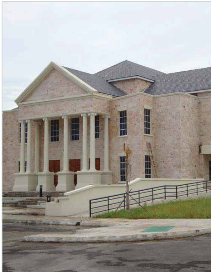
The Port Antonio Courthouse completed in 2008
