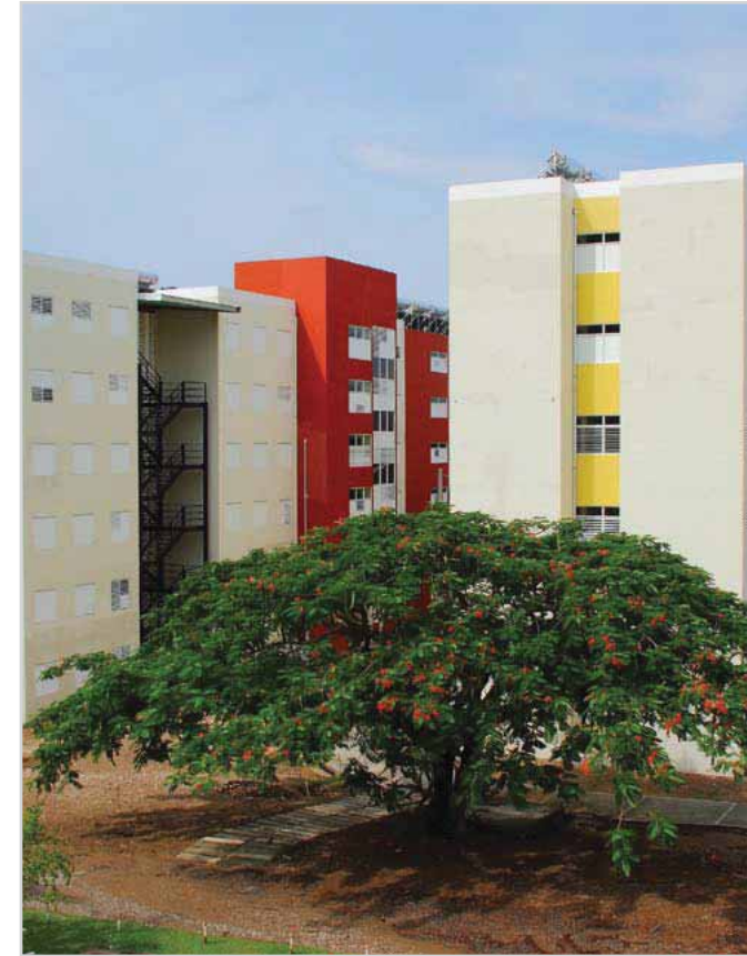
University of the West Indies Student Housing completed in 2012
