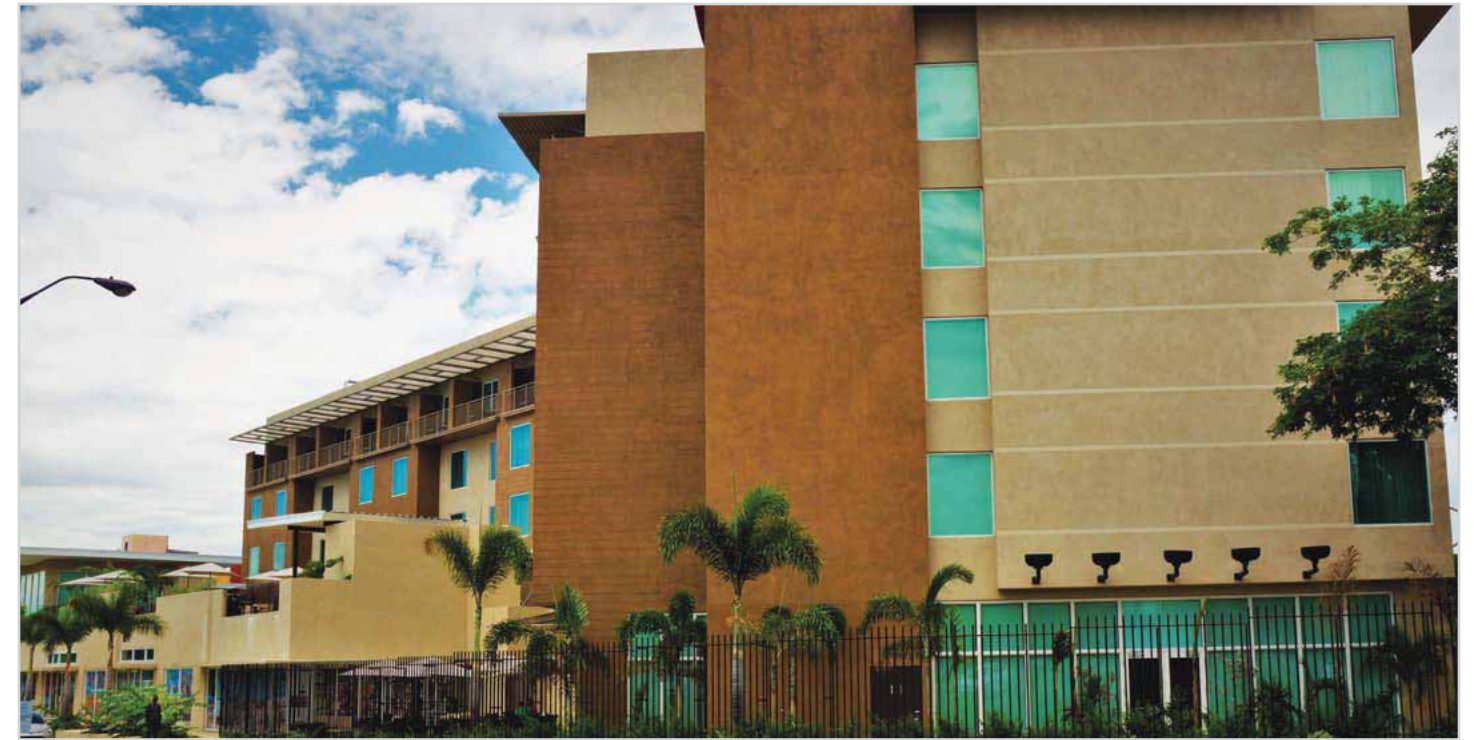
The Courtyard by Marriott completed in 2015
